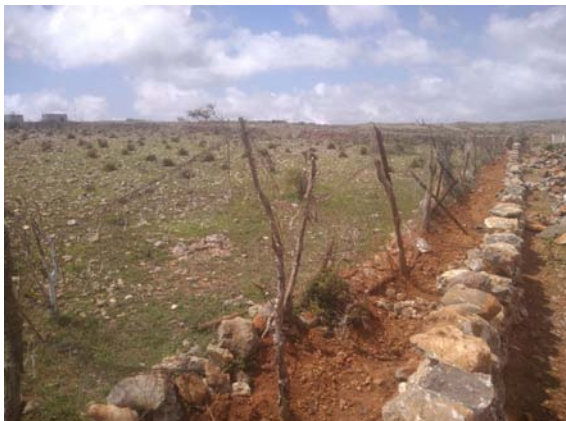
A new stony wall was built surrounding the old broken fence in Ras Ayre village where young dragon's blood trees have been grown since 2006. Thanks to the new wall (supported by the Frankinia project and by Eva Zubeck's donation, and constructed by the Keybani family), Boswellia dioscoridis and Boswellia ameero seedlings will be planted here among young dragon's blood trees (photo by Salem Keybani).
